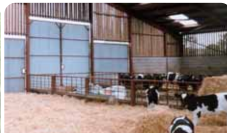
at Cattle shed
