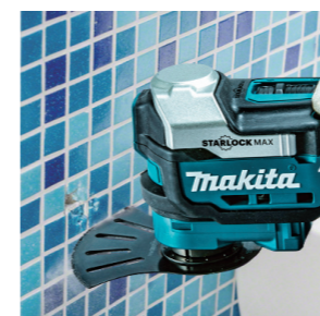
Routing joints on wall tiles
