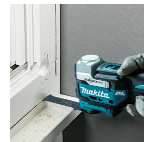
Removal of window frame
